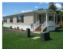
Modular Home - factory built & set on frost protected foundation - falls under International Building and Energy Conservation Codes
